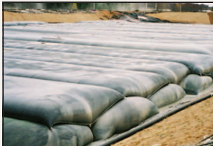
Geotube® containers in activated sludge basin at paper plant.
