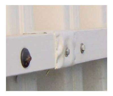
Finally, after your retaining structure is complete, it is a good practice to periodically check back to make sure that everything is aging as expected and no maintenance is required. Though the metals used are designed for marine environments, all metals corrode eventually. You should make sure that no premature corrosion is taking place, and if found, the corroded material should be removed and sealed to prevent damage to the integrity of the structure.
