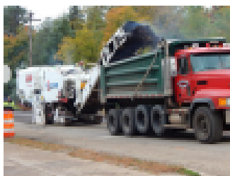
Milling of the surface layer
